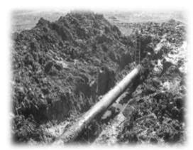
Wax buildup causes pipeline throughput to slow down. To prevent storage tanks overflow, some wells have to be shut-in or choked down. The operator does pigging to maintain pipeline ID, but it quite often happens that the pig gets stuck. It leads to days of downtime, using alternative route to terminal by trucks and oil sales lost. To fix it operator does either reverse circulation to send the pig back or excavation works to expose pipeline. Excavation in wet part of the pipeline is impossible.
